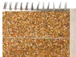
Pebble Vibracrete Wall with Spikes
