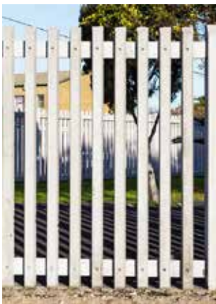
Palisade Fencing 2.4m high
