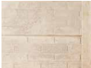
Brick Line Vibracrete wall
