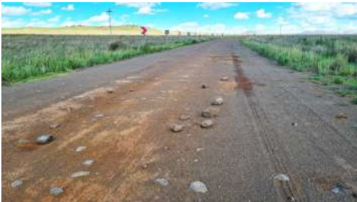
Loose gravel and rock pebbles in the form of a windrow between vehicle tracks ( right ) and large rocks in the road ( top )
