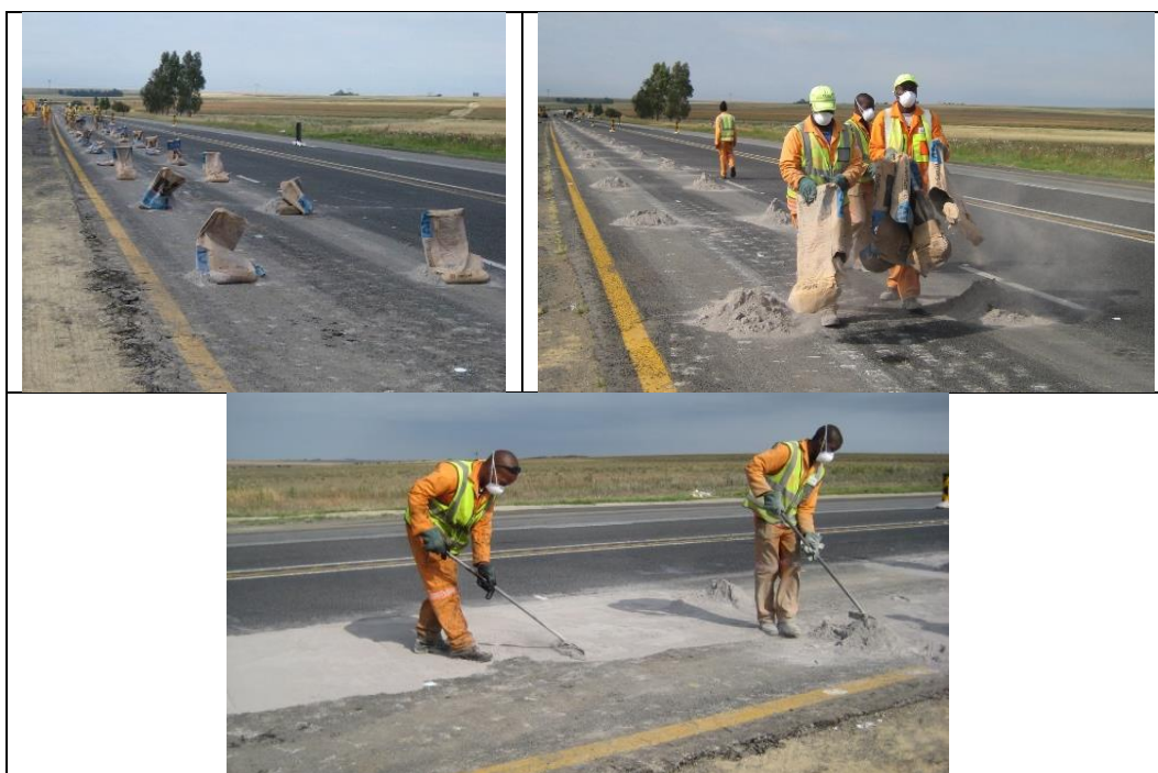
Figure 17. Spreading Cement to be Mixed into Recycled Materials
