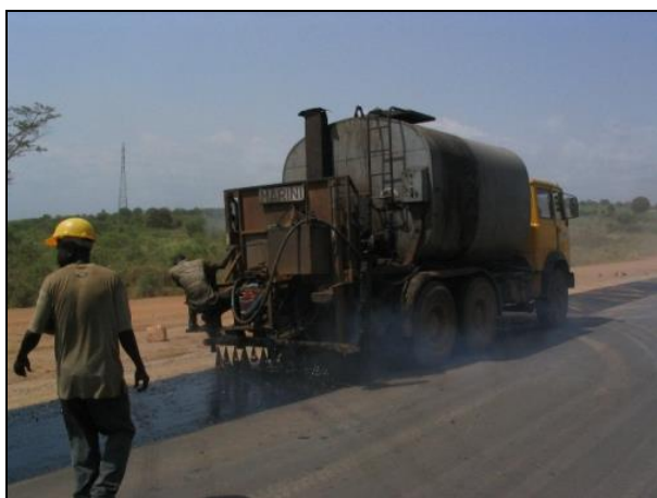
Figure 15. Application of a Tack Coat
