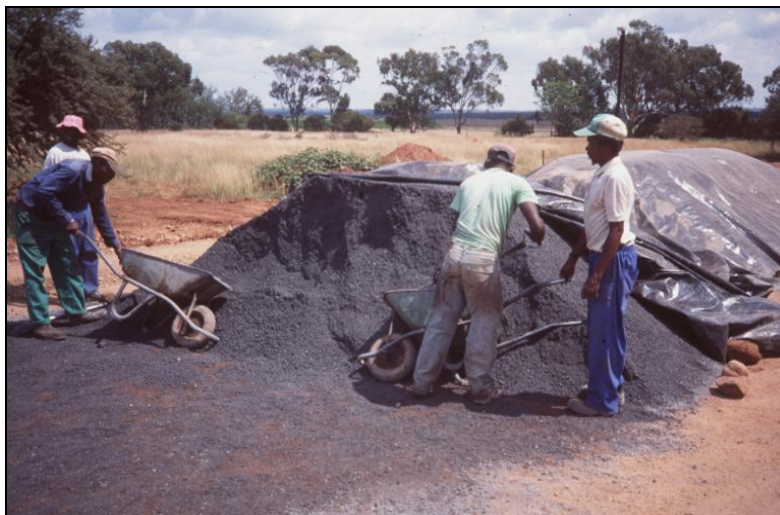
Figure 23. Ash, Used to Construct Pavement near Cullinan, Gauteng
